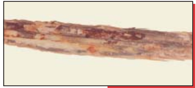
Close-up (25X) of UNPROTECTED scribe(scratch) showing pitting, metal loss & severe corrosion
